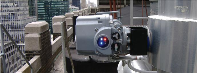
The HQ series electric actuator boasts being both small and lightweight while still producing high torque output. As the smallest member of the HQ series, the HQ-004 weighs only 2.6lbs(1.3kg), but is able to produce 350 in-lbs(40 N-m) of torque. Providing similar size-to-torque efficiency, the HQ series offers actuators producing over 34,500 in-lbs(3,920 N-m) of torque.
